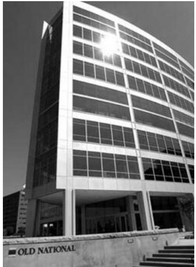
Old National's $47 million headquarters building on the riverfront in downtown Evansville opened in October 2004.
