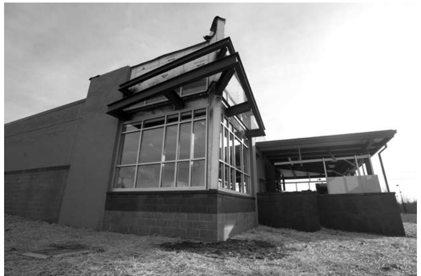
Ceramics Center in later construction phase. The facility opens in January.
